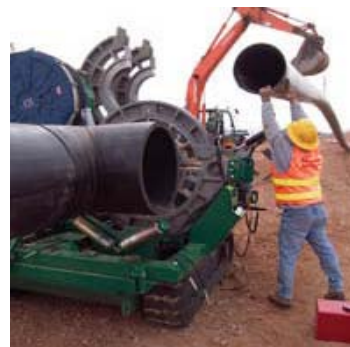
HDPE pipe sections are fused together to create a leak-free system.
