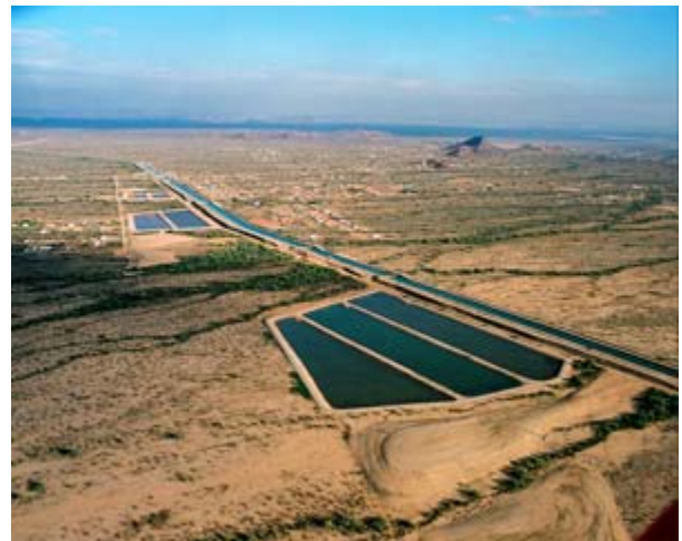
There are 19 basins in the Tonopah Desert Recharge Project, which covers a total of 542 acres, 40 miles west of Phoenix.
