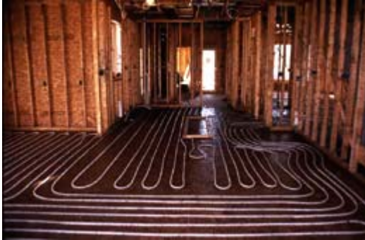
PEX Tubing Layout on Floor for Radiant Heating
