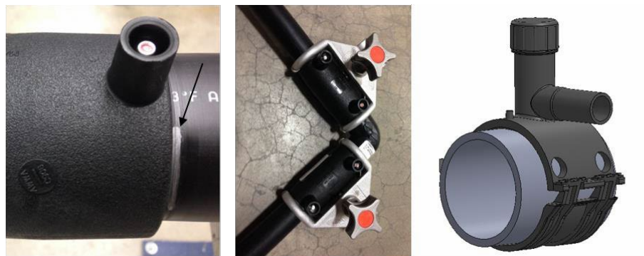
Stab depth is correct
