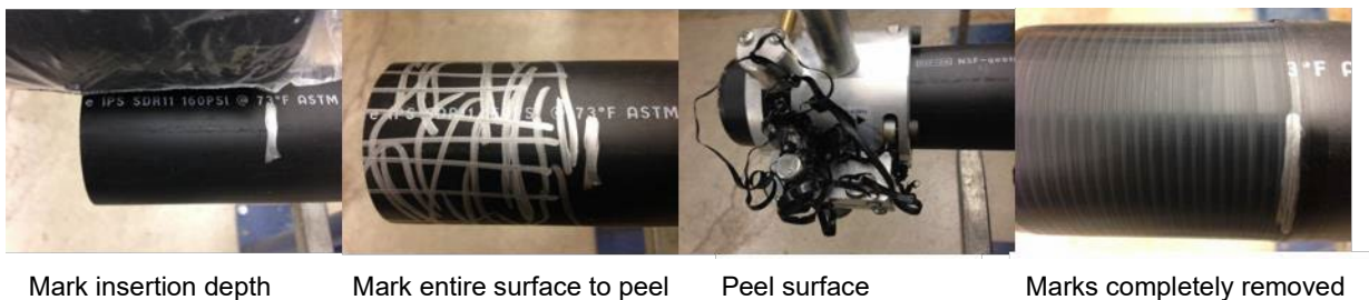
Figure X-o - Correct Peeling
