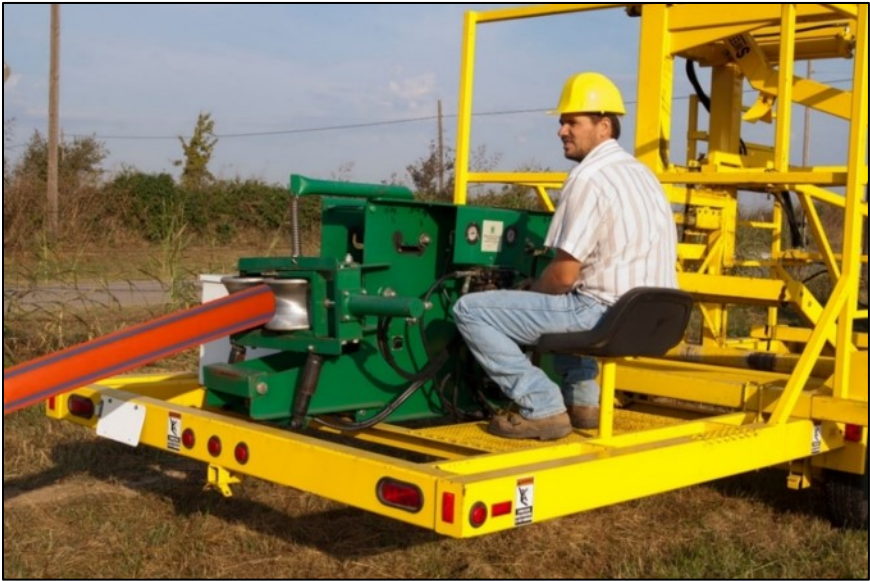
Figure 15: Nominal 6 inch coiled conduit being pulled through a re-rounding device
