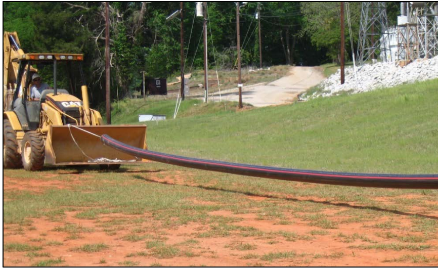
Figure 10: Example of a Straightening conduit by allowing it to lay flat
