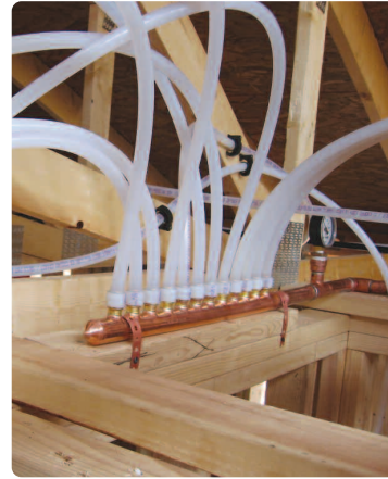
Uponor’s brass manifolds in combination with their ProPEX fittings offer a durable, leak-resistant plumbing and fire protection system.
