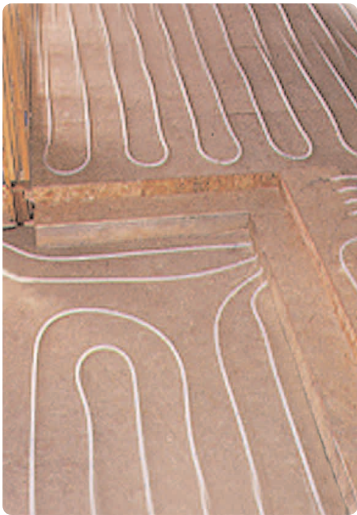
Uponor's Wirsbo hePEX™ plus tubing was installed over suspended wood floors and covered with a poured underlayment on the first and second stories of the home.
