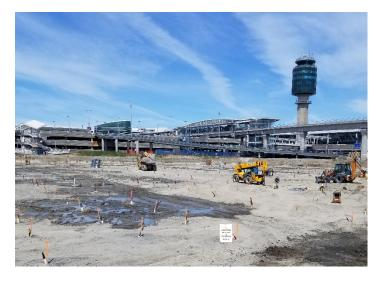
Each 500-foot borehole contains 1,000 feet of 1 1/4-inch PE4710 HDPE pipe. These pipes link to lateral headers that carry the fluid to the Central Utilities Building. The headers feed into manifolds that tie into heat pumps, which distribute the geothermal energy to and from airport buildings. Ground Source Energy used 16,800 feet (5,120 m) of 1 1/4-inch PE4710 HDPE header pipes to complete the geoexchange system. "There's pipe everywhere," said Mooney.
