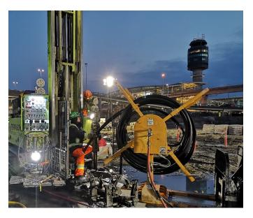
Borehole drilling and installation of the geothermal loops and headers is complete, and the 67,000 square foot (6,230 square meter) Central Utilities Building (CUB) is expected to be operational by 2022.
