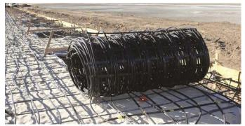
Fabricated mats of PEX pipe were delivered to the project and numbered to correspond with the design for connection to the correct manifolds.
