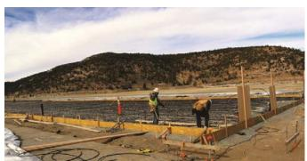
Some 22,500 linear feet of Viega PEX Barrier tubing was installed in less than one day using Viega Climate Mat.
