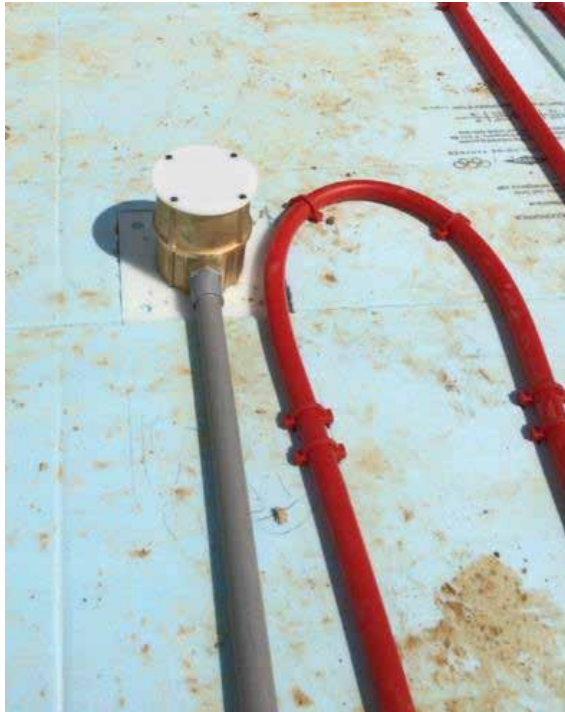
Sensor socket before concrete
