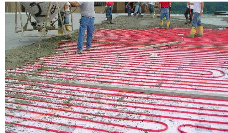
Right: Medivac landing pad on hospital rooftop
