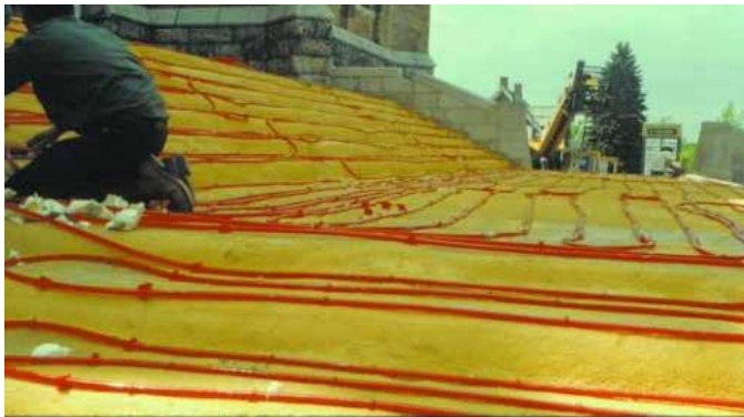
Left: Spray-foam insulation on old stone steps (church)
