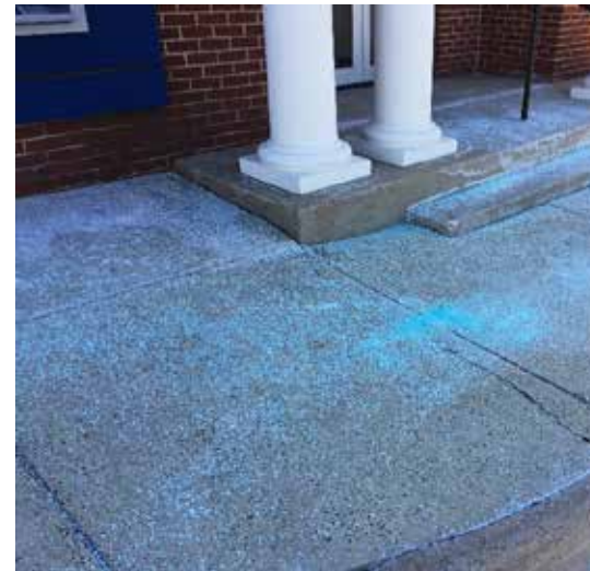
Right: Salt at building entrances
