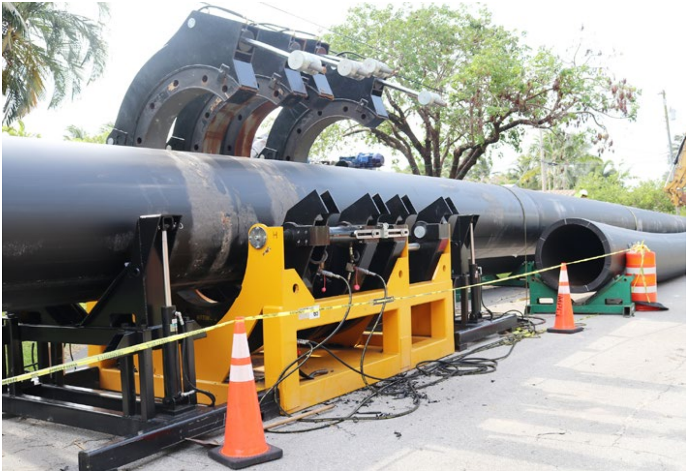
HDPE's heat-fused joints create a leak free, self-restraint, monolithic piping system
