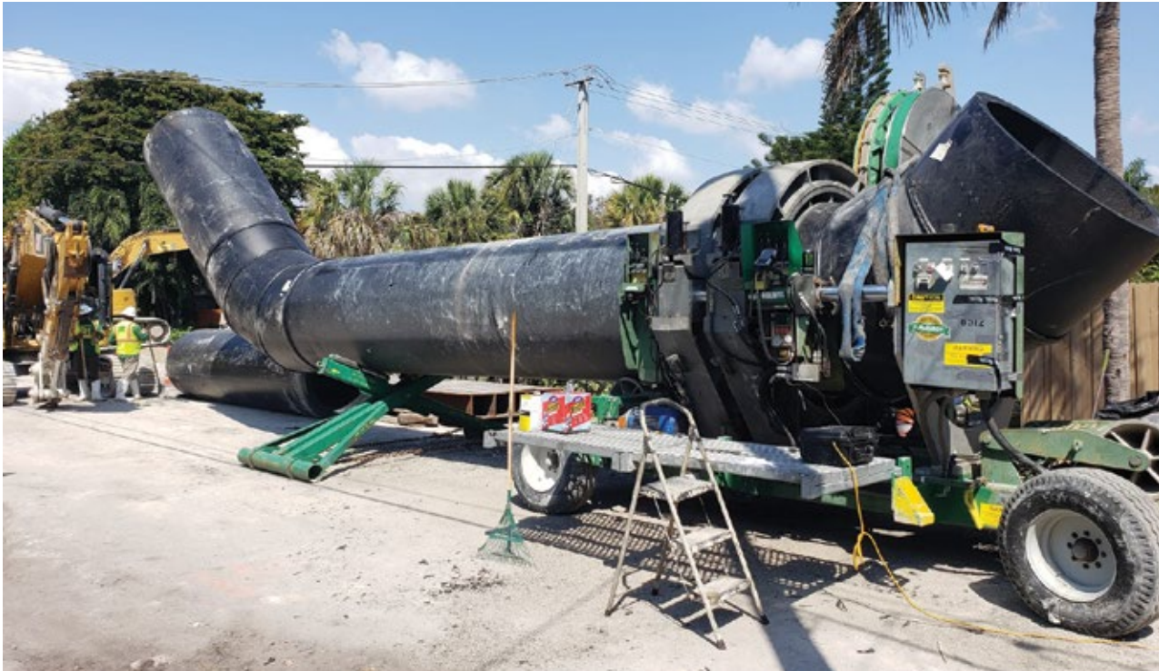
Fused joints eliminate infiltration and exfiltration
