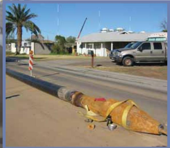
At left: AUI Sewer saddle fused to 14 inch HDPE. Above right: 14 inch Bursting Head Assembly with 14 Inch HDPE dr 17 pipe attached
