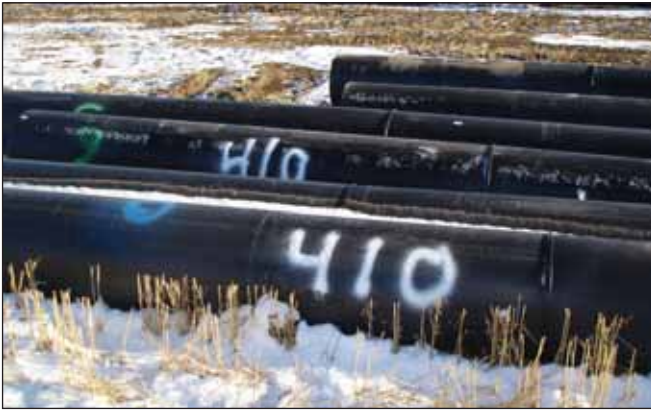
Welded 18" O.D. HDPE.
