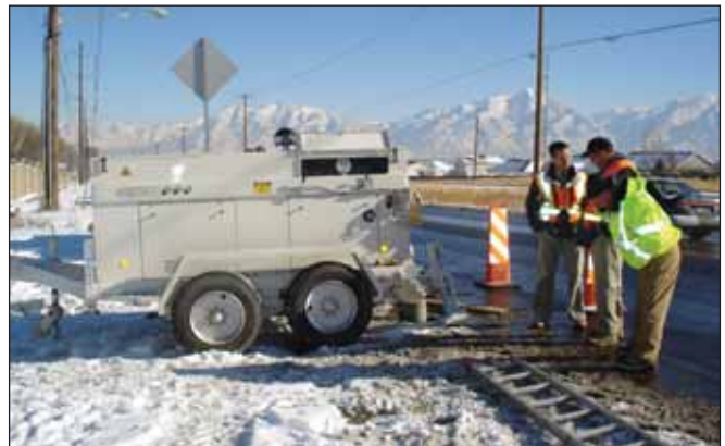
TT Technologies Grundoburst® with PEC Engineer and Noland and Sons.
