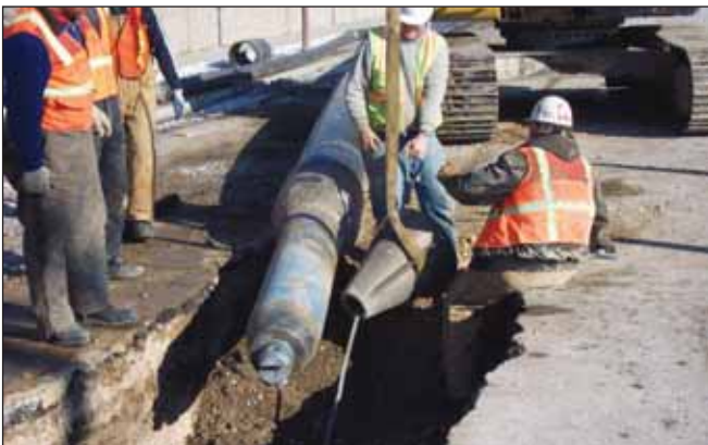
Noland and Sons installing splitter on bursting head.
