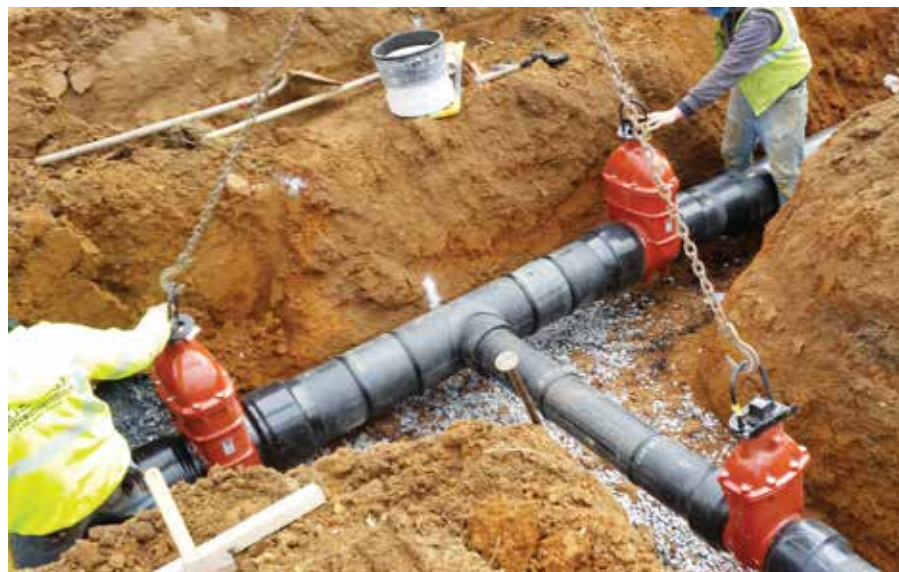
When disinfecting an HDPE potable waterline, it is important that purging applies to distribution mains as well as each service line and service connection.
