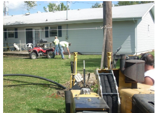
The City of Princeton is helping the environment while protecting its citizens. Putting overhead utility lines underground using HDPE conduit pipe reduces the need for the more than 800,000 wooden poles purchased by electric companies annually in the United States.
