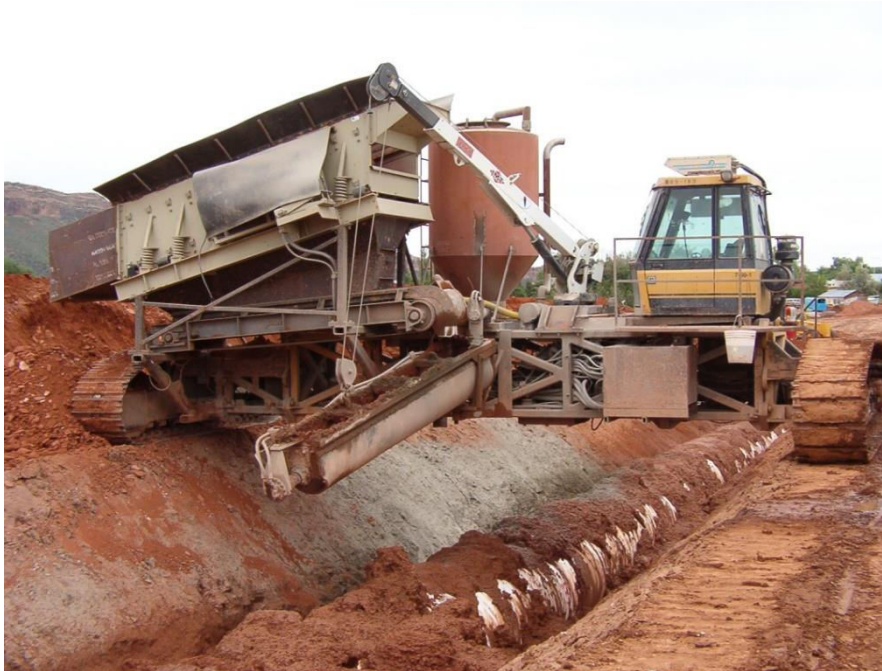
Figure 6 Flowable Fill Placement Operation
