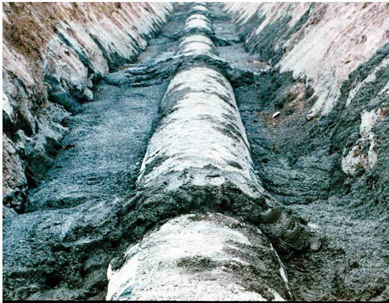
Figure 1 Trench Filler Flowable Fill
