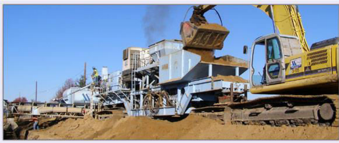
Figure 4 Insitu Soil Mixing Equipment
