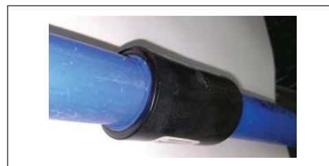
Fig. 13 Service Line Socket Fusion
