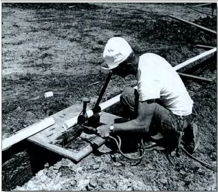
Figure 1: Natural Color Polyethylene Pipe being Fused, 1959, in Caney, Kansas
