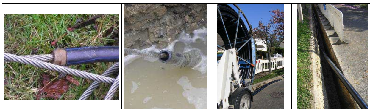
Figure VI: Examples of pipe installation during the trials
