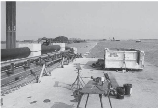
**Figure 4** PE Pipe Weighted and Floated for Marine Installation
