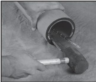
Figure 19 Install Split Ring Stiffener in PE pipe
