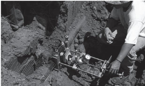
**Figure 3** Saddle Fusion Repair
