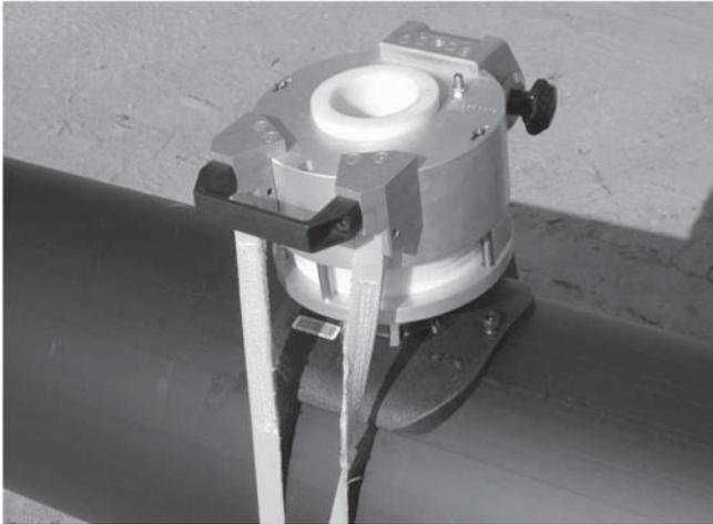
**Figure 4** Electrofusion Patch Repair
