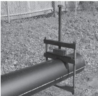
**Figure 15** Mechanical Re-Rounding Clamp Installed
