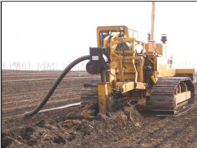
With the advent of HDPE resin and the ability to make corrugated pipe, the ag market became the starting point of more pipe development. In less than one generation, corrugated HDPE pipe displaced a product that
