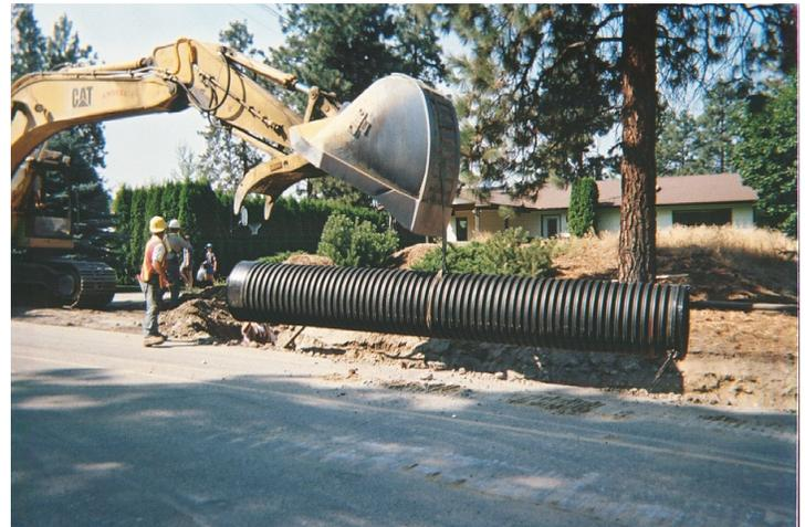
Easy to move, more than 400 meters of HDPE pipe was used for a water drainage upgrade project here.
