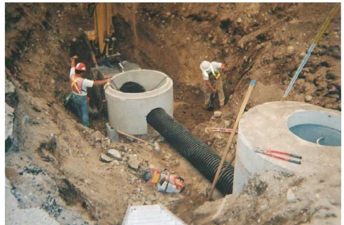
A two-man crew quickly positioned BOSS 2000 HDPE pipe for the ditch in-fill project.
