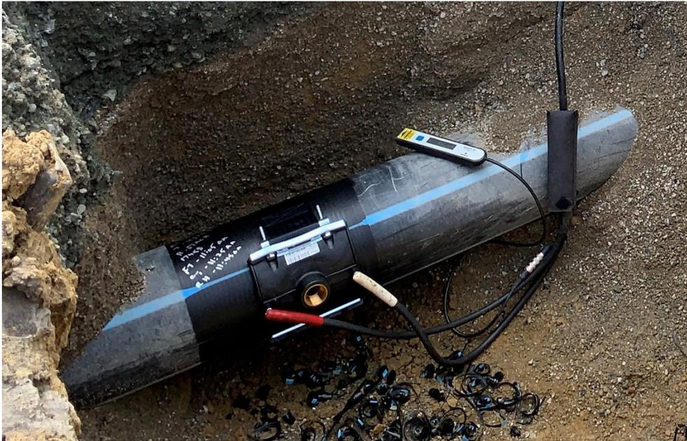
Information about electrofusing large diameter polyethylene pipe can be found in *MAB Generic Electrofusion Procedure for Field Joining of 14 inch to 30 Inch Polyethylene (PE) Pipe (MAB-02-2017)*, one of two electrofusion documents available for free on the PPI website [www.plasticpipe.org](http://www.plasticpipe.org).
