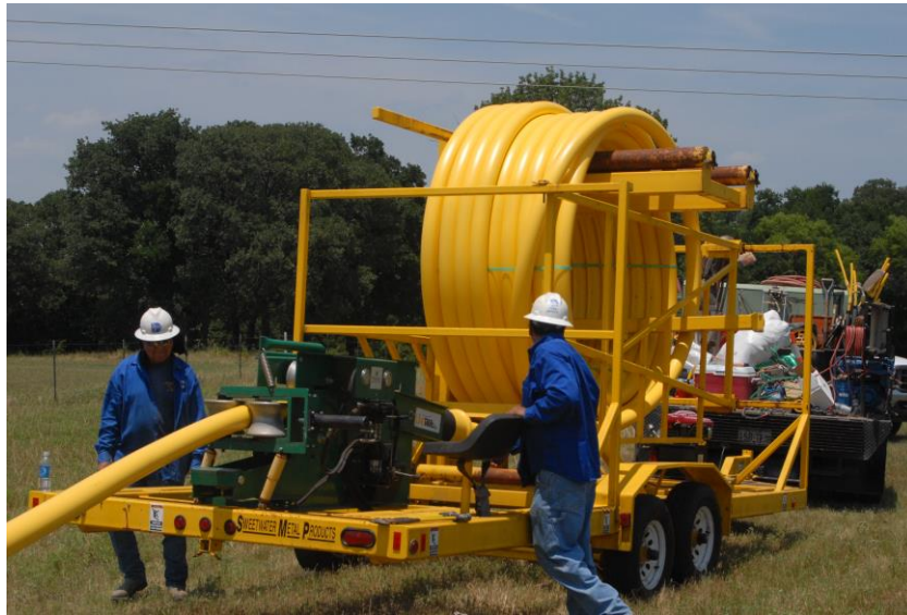
PPI DSC 0839: MDPE pipe for gas distribution
