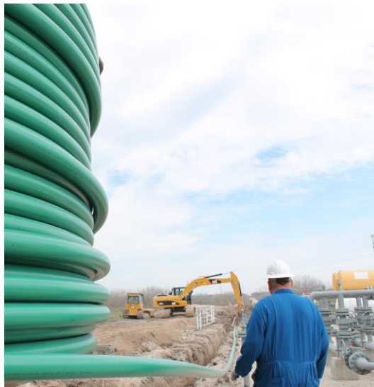
PPI DSC 0839: MDPE pipe for gas distribution
