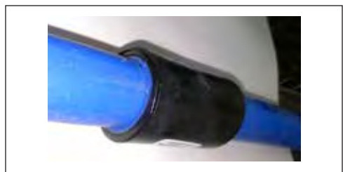
Fig. 13 Service Line Socket Fusion
