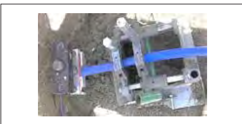
Fig. 12 Service Butt Fusion
