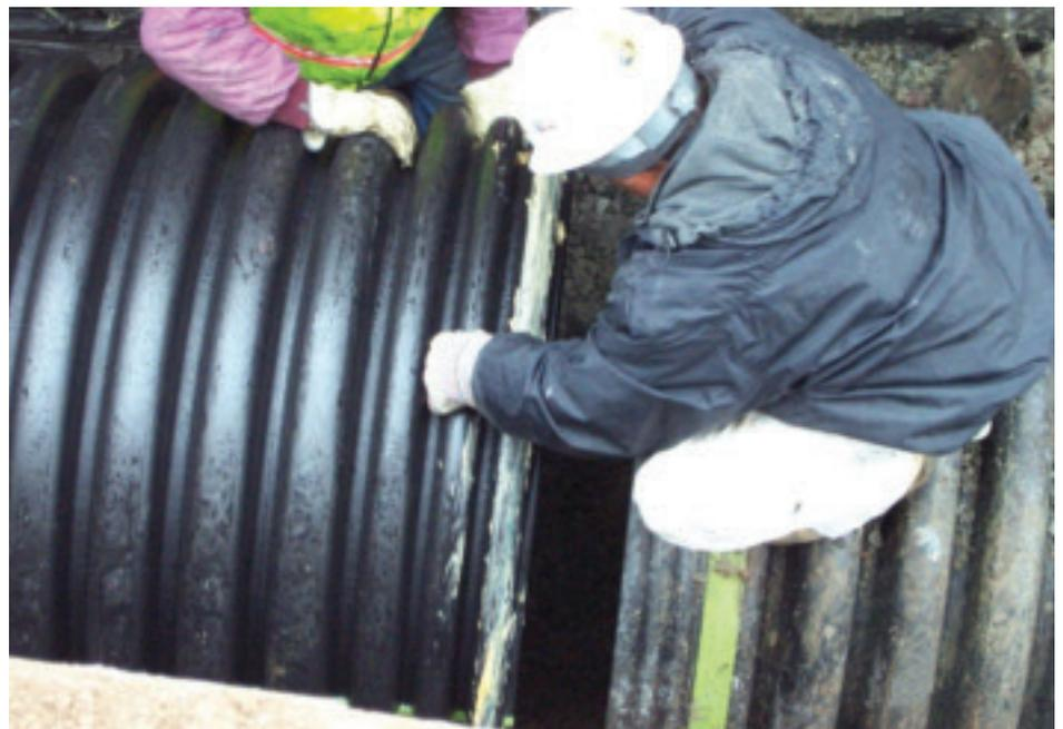
were constructed to the centerline of the road. The second phase installed the trunk line down the middle of the northbound lane and the continuation of the cross pipes in order to connect to the trunk line. This required the manufacturing of non-standard lengths of pipe.”
