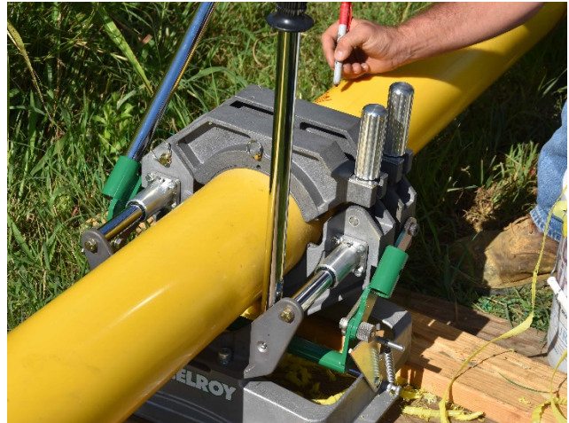
Fusing sections of PA12 pipe
