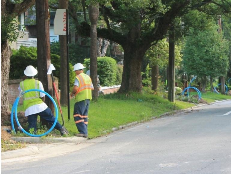
With heat-fused joints and service saddles, tees and other connections, HDPE pipe is also corrosion resistant, does not promote tuberculation, and can be installed using cut-and-cover and trenchless methods to replace old lead water pipe. The Plastics Pipe Institute offers resources to evaluate the HDPE pipe alternative.
